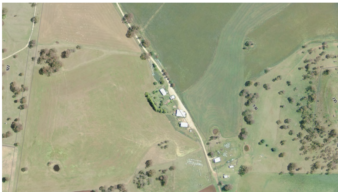
Figure 4 – Showing building encroachments over boundary
